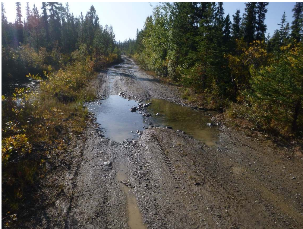
Photo 1. Water flowing over the road at Site 0 from the pond on the left (east) to the creek on the right (west).
