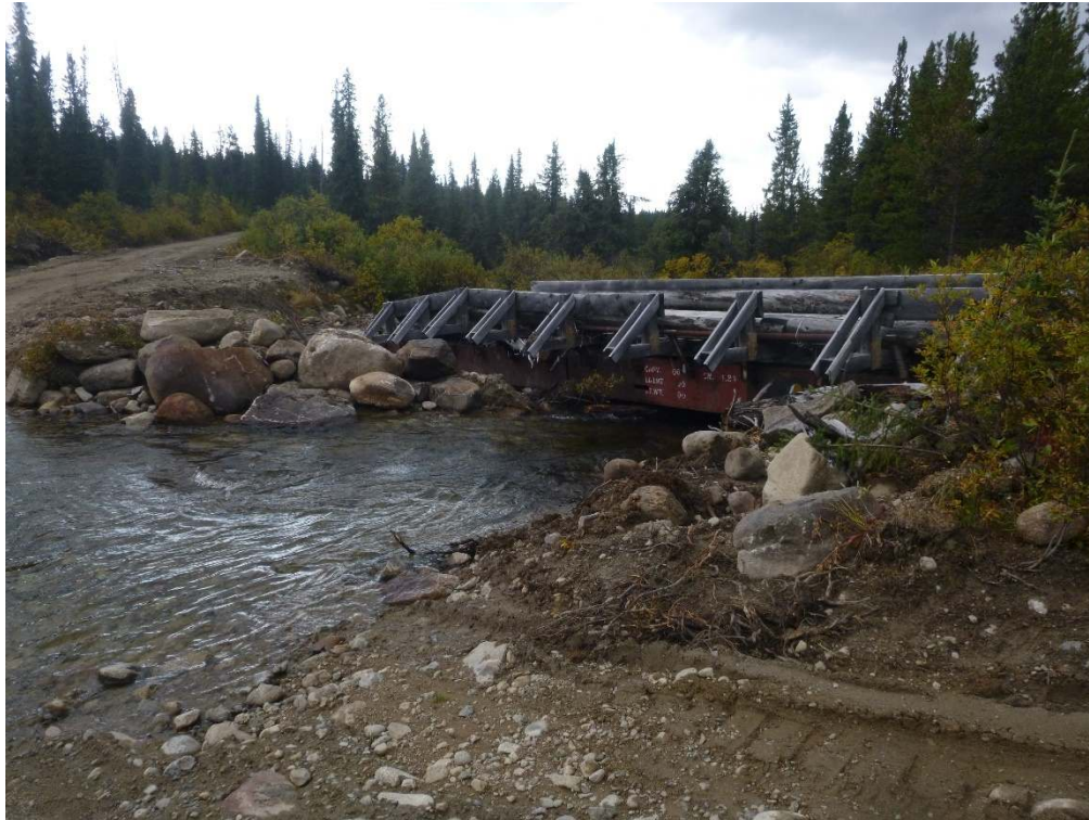
Photo 20. The washed-out bridge at Site 5 just downstream of the ford crossing.
