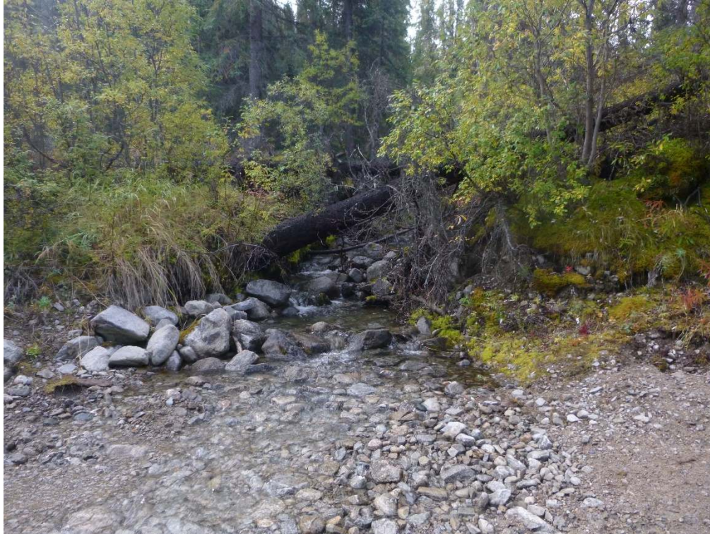
Photo 29. Upstream view of the creek flowing onto the road at Site 10.
