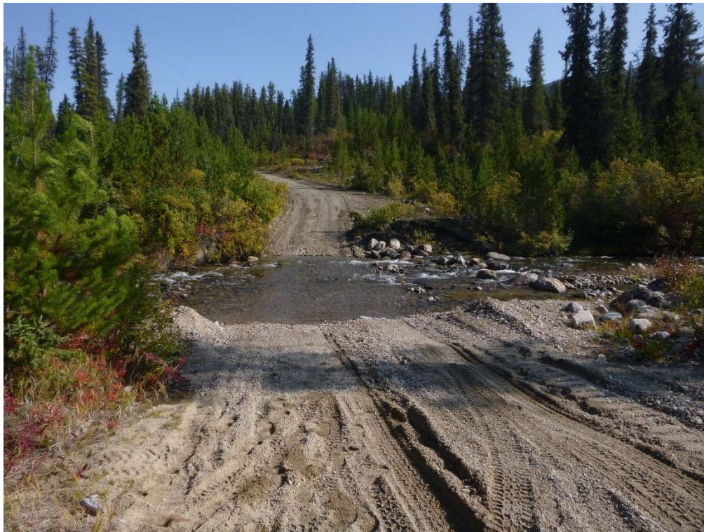
Photo 24. The crossing at Site 9 looking north.
